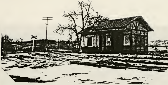
Fig. 73 Anselma Station and surrounding landscape, 1937. Photograph Collection, Railroad Stations - West Pkkeland Township - Anselma, Chester County Historical Society, West Chester, PA.
